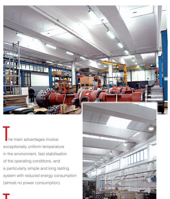
he Duck Uap radiant panels are produced in 6 different models, with 2 standard colours, and others upon request. Each model features elements measuring 4 and 6 metres in length (3 and 5 metres upon request).
